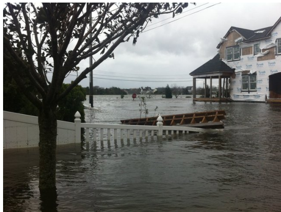
(a) Water damage: flood from the bay
